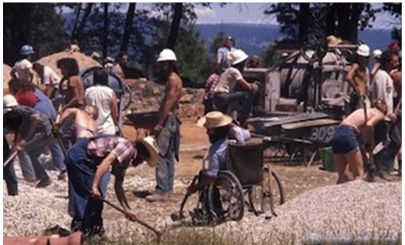
Construction of Oak Tree School
